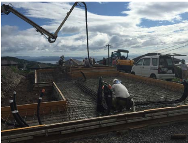
Construction of the Beppu geothermal power plant
