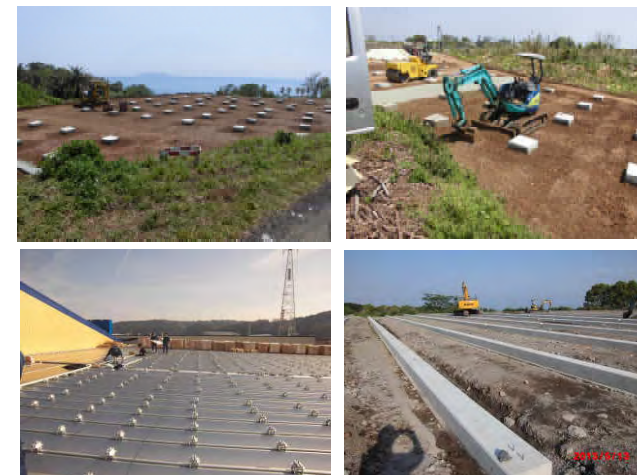
An image of the start of construction on-site (contracted )
